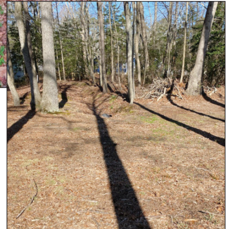
Clogging drainage ditches – Illegal dumping of leaves and yard debris into drainage ditches and placing debris on the golf course.
