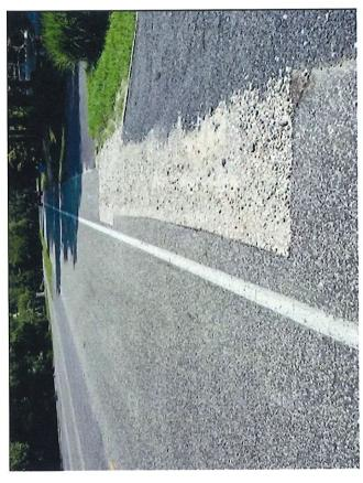
REMOVE PINE NEEDLES, WEEDS, BLUE REFLECTORS FILL HOLES/PAVE HOLES LEFT BY UTILITY WORK to allow full width of shoulder
