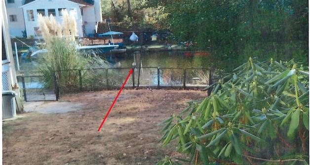
200.5.B.3. - The enclosure shall not be constructed of metal posts, metal rails, or wire mesh. The metal fencing must be removed asap.
