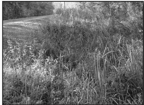
A wide, shallow drainage area can reduce erosion and control sediments. Photo by Bruce Nichols, NRCS
